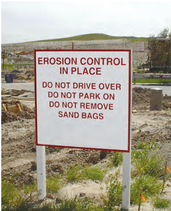
Figure 4. Use signage to help educate construction staff.
