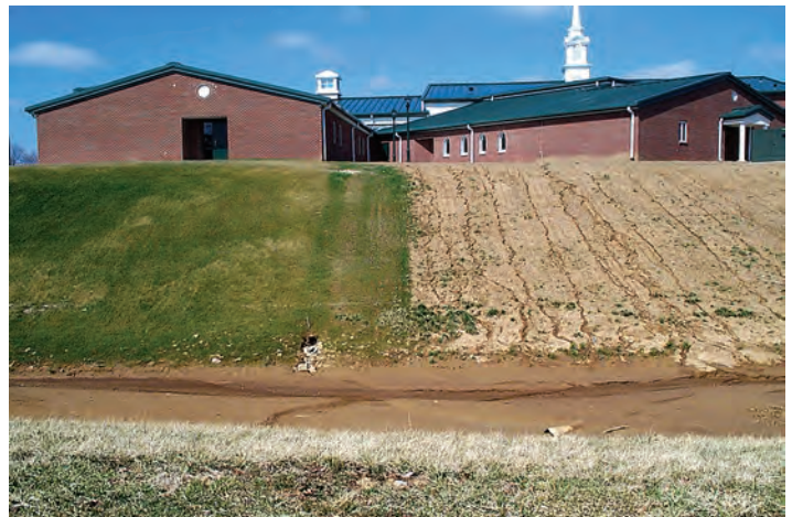
Figure 16. Seeding is an effective BMP that can be used to temporarily or permanently stabilize disturbed areas.
