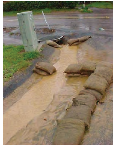
Figure 5. Make sure storm drain inlets are protected.
